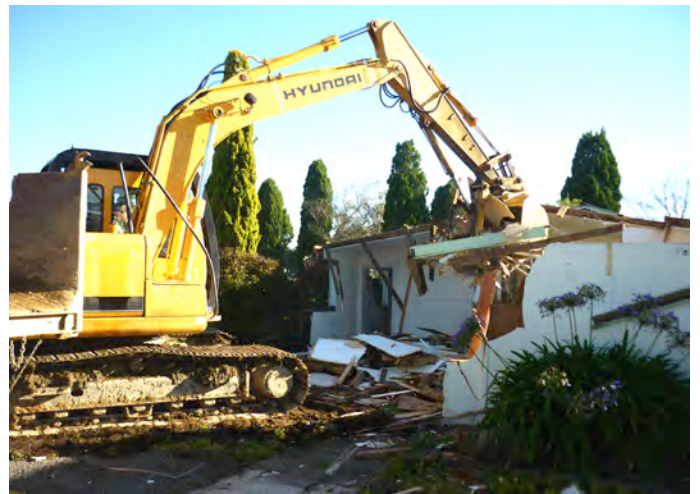
Demolitioning the old accommodation/utilities block
